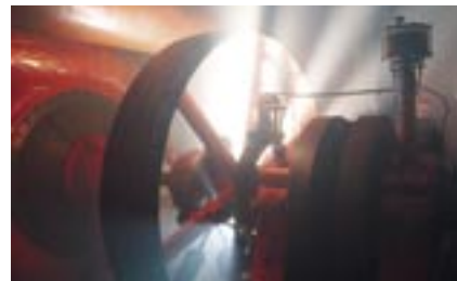
Station de pompage Craig - Montréal - 2004
